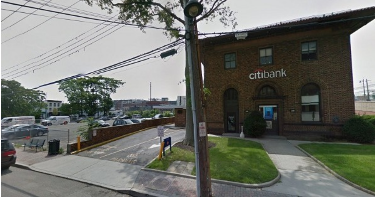
Redevelopment site at 199 2nd St. Mineola / Google Maps image
